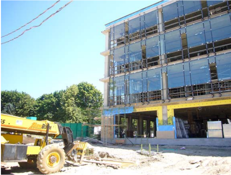
The Queen Street West face of CAMH's construction
