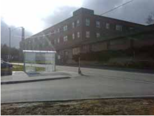
Nicholls Building, Peterborough
